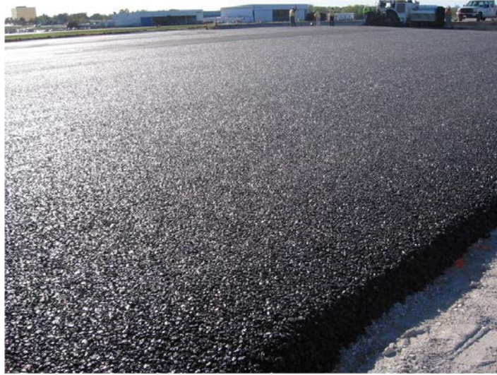
Figure 9.12. Completed porous asphalt installation.
