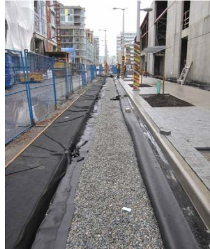
Figure 9.2. In-place geomembrane (geotextile ready to be folded to enclose the shoulder).
