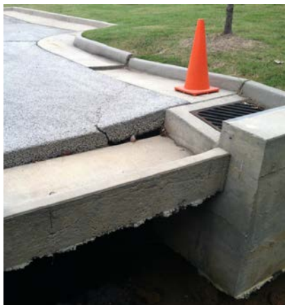
Figure 9.15. Pavement failure due to water erosion.
