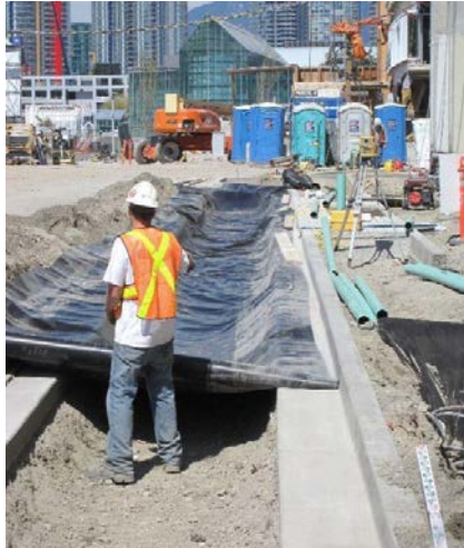
Figure 9.1. Installation of a geomembrane.
