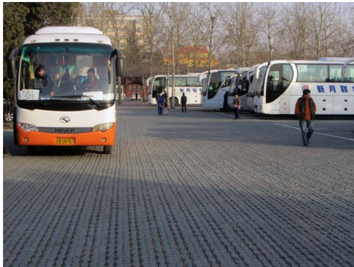
Figure 3.1. Turf pavers providing structural support and vegetative growth/permeability.
