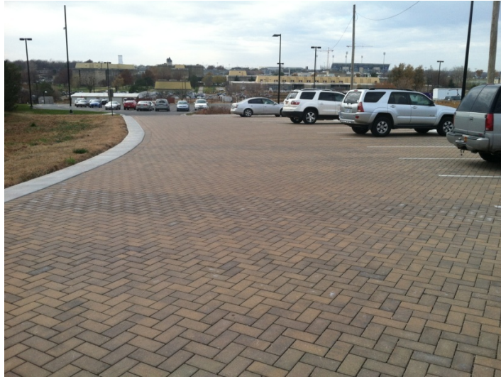
Figure 9.14. Typical permeable interlocking concrete pavement installation.
