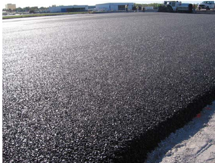
Figure 3.3. Porous asphalt pavement.
