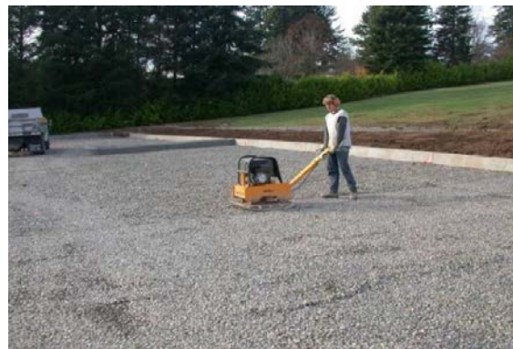
Figure 9.8. Inappropriate (too small for size of project) for compaction.
