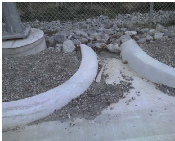
Figure 9.6. Example of a curb cut-out.
