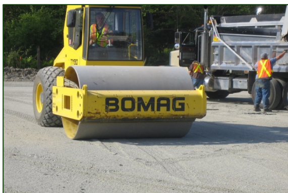
Figure 9.7. Appropriate compaction equipment for open graded aggregate.
