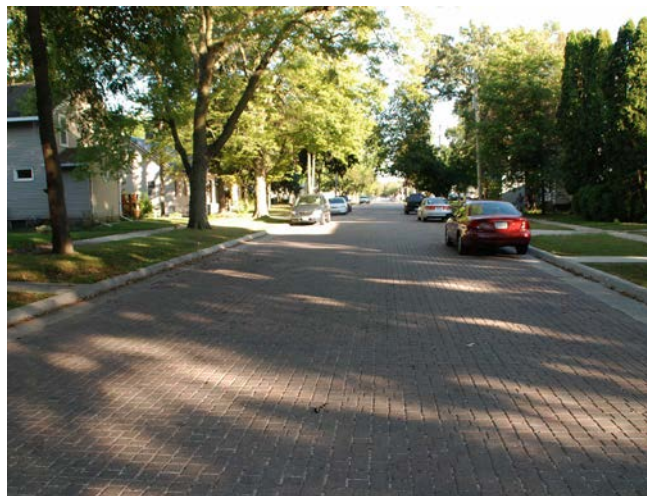
Figure 3.5. Permeable interlocking concrete pavement.
