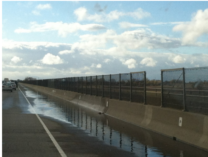
Figure 1.1. Ponding on highway shoulder.
